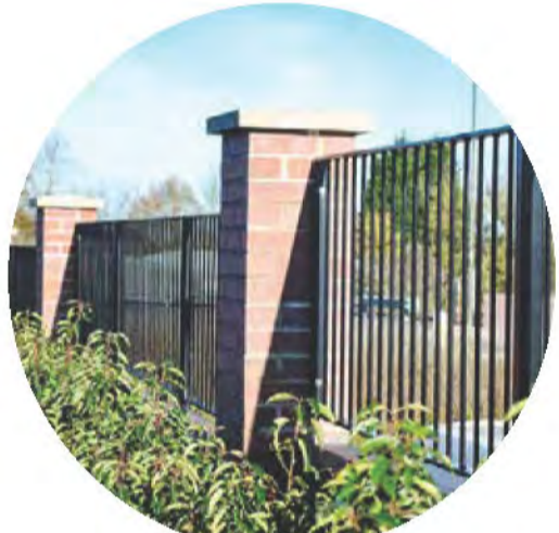
Boundary Wall & Railing
